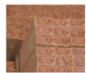
Profile boards / Basic Construction
